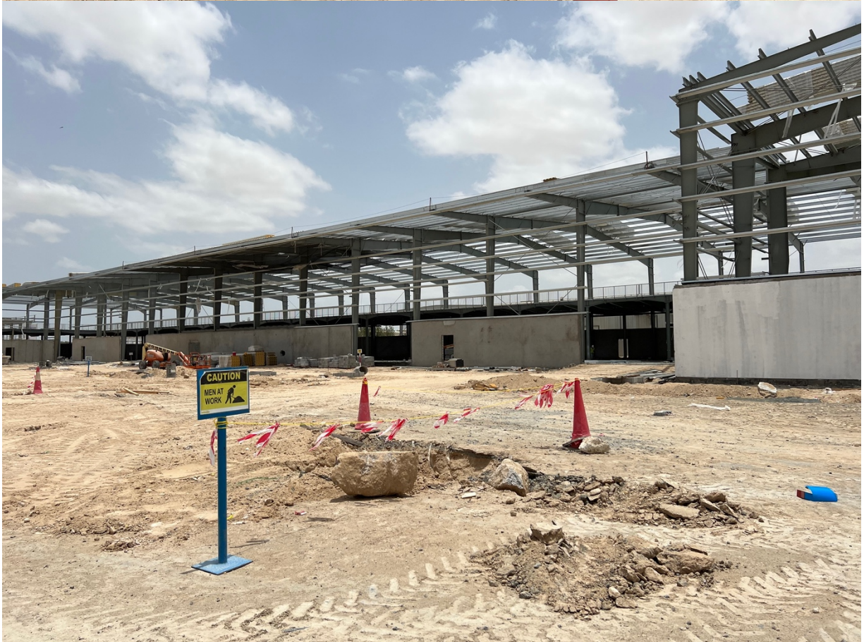
AL FARES WAREHOUSE 5
